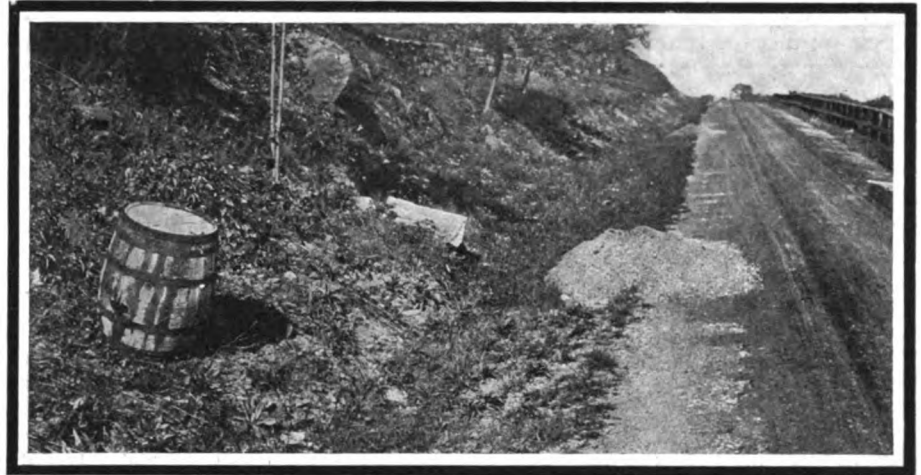
Material for resurfacing and barrels of oil are distributed along patrolled highways in New York
